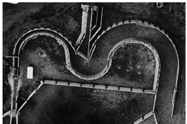
Fig. 2. This design is for loading livestock. The cattle walk in a single file line and the ramp width is 30 inches. (Reprinted with permission from the Temple Grandin website)
